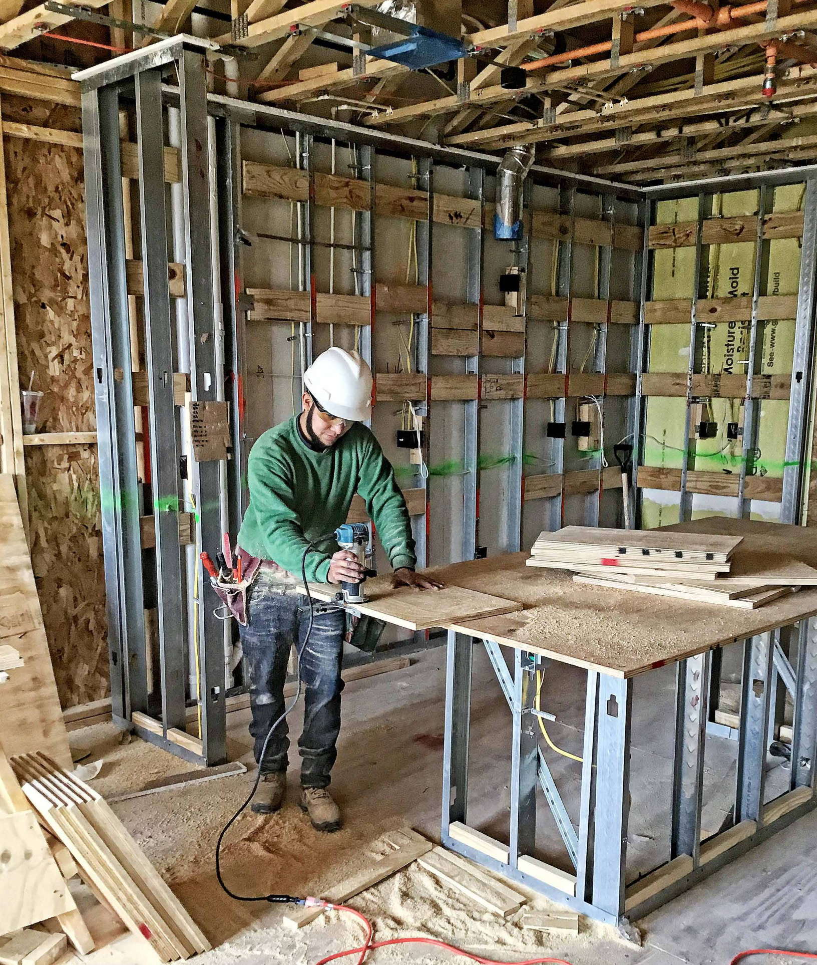
Holmes Beverly construction
