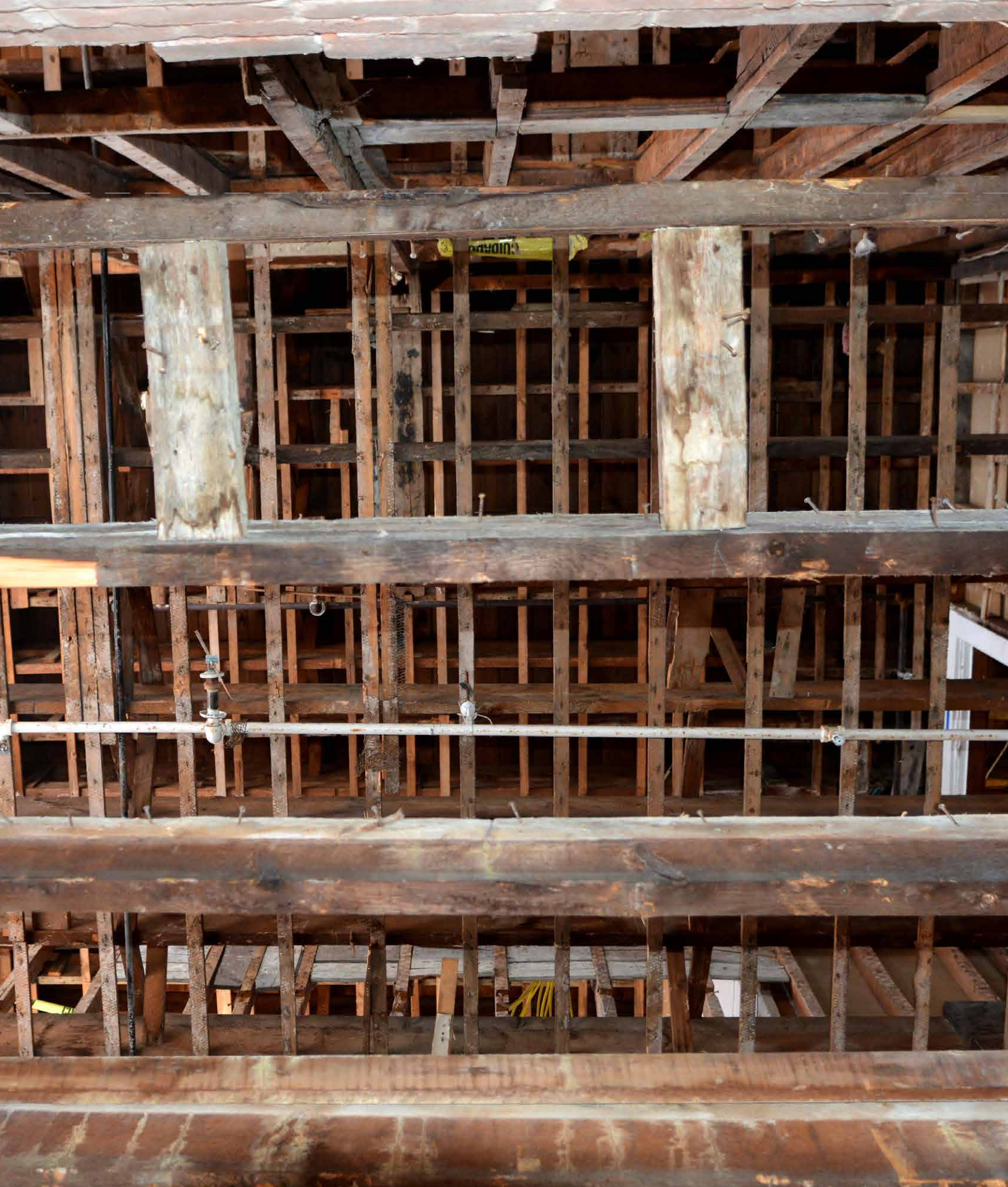
Demo underway at Abby's House, Worcester
